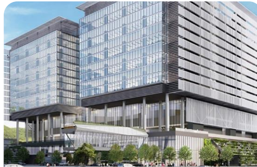
Advanced Manufacturing Centre – Electro-chlorination System
