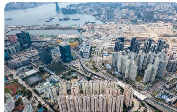
Kai Tak Residential Development
