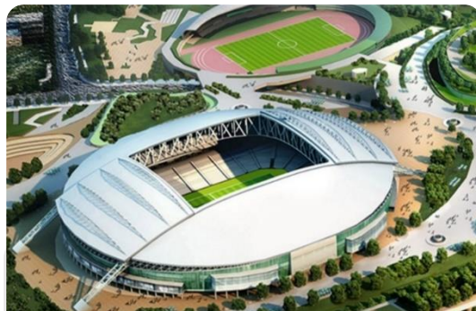
Kai Tak Sports Park – Building Materials
