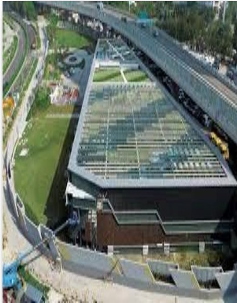
Additional DCS at Kai Tak – Sea Water Electro-chlorination System
