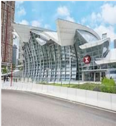
Express Rail Link – West Kowloon Station
