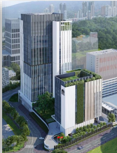
District Court at Caroline Hill Road
