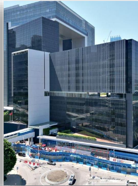
Expansion Project of the Legislative Council Complex
