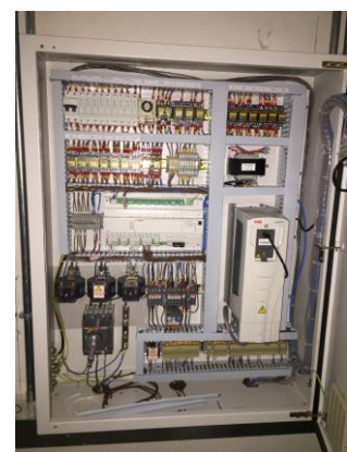
Variable Speed Drives for PAUs
